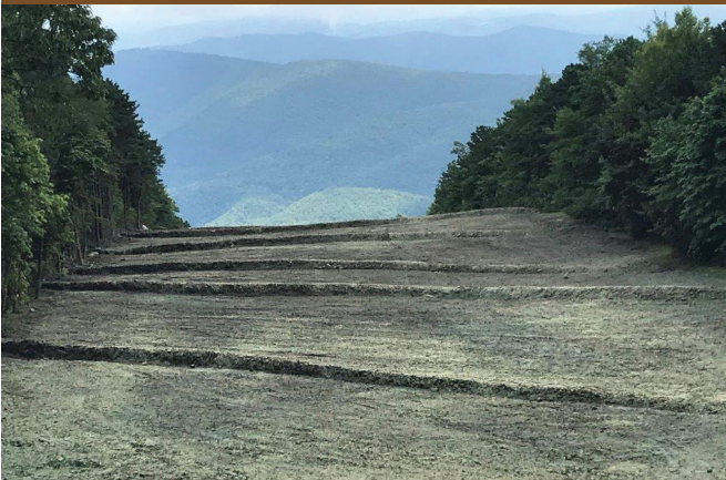
Energy / Pipeline Restoration
